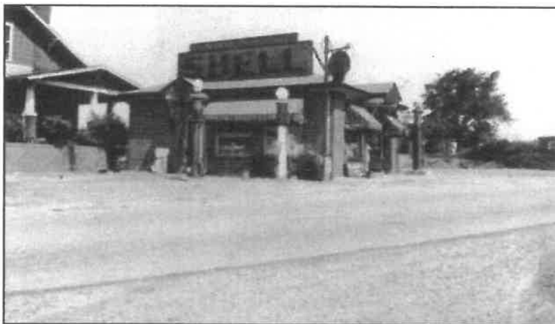
Quality Oil Company, R.L. Moser Shell Service Station at Ogburn Station, Courtesy of Forsyth County Photograph Collection
